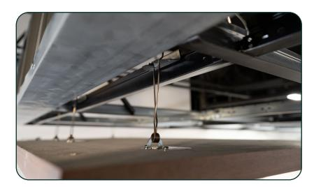
Once all springs are secure, gently raise the panel one side at a time until panel is pulled into place.
